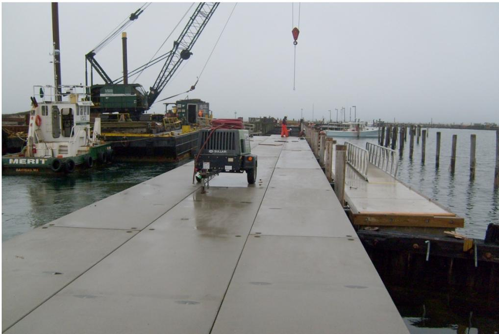
Town of Chilmark honored marine contractor C.White Marine for replacing burned timber pier on Menemsha Harbor with concrete and steel construction. Work was completed in record time during challenging weather. Photo is showing concrete deck plank installation. Finished pier is 15 feet wide and 500 feet long.
